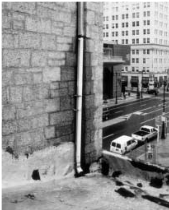
Check gutters and downspouts during, or just after, a rain for water overflow and loose connections.
