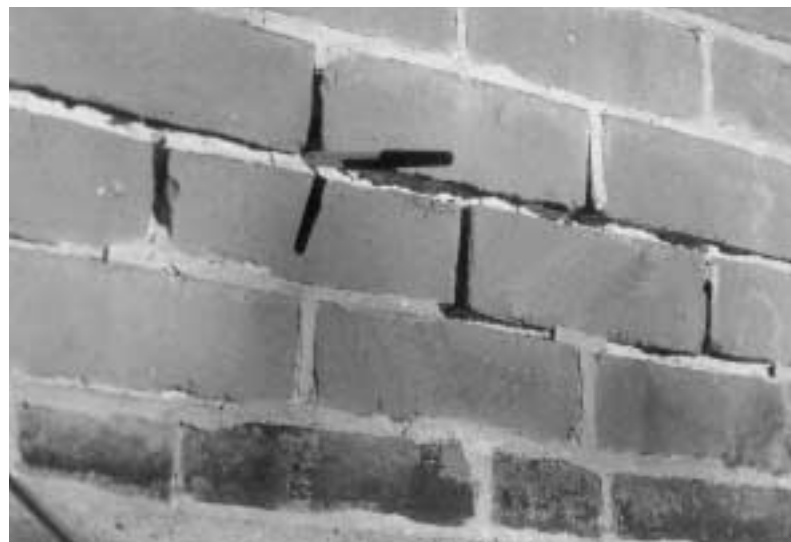
Repoint open and deteriorated mortar joints with new lime mortar in a color and texture to match the original mortar.
