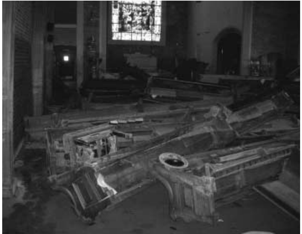
St. Paul's Episcopal Church and School in New Orleans suffered extensive flood damage, including significant mold growth on these overturned pews.
